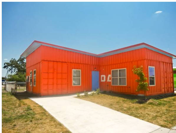
A house built using three 45-foot shipping containers is part of a comparable study on energy efficiency funded by the Neighborhood Stabilization Program (Photo: SAAHC)
