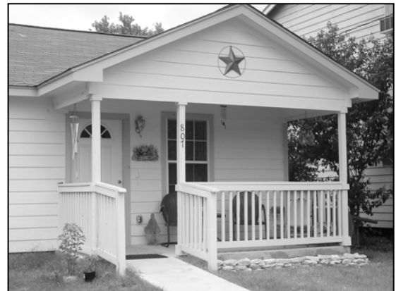
Above: This home in Lockhart became wheelchair accessible at its front entrance as part of its rehabilitation through the HOME Program's Owner Occupied Assistance.
