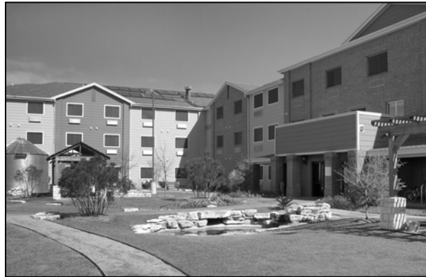
Above: A Multifamily Bond development, Spring Terrace in Austin is a Single-Room-Occupancy complex that has “green” features such as solar panels and a rain collector.
