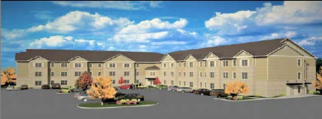
TYPICAL BUILDING ELEVATION/PHOTO
